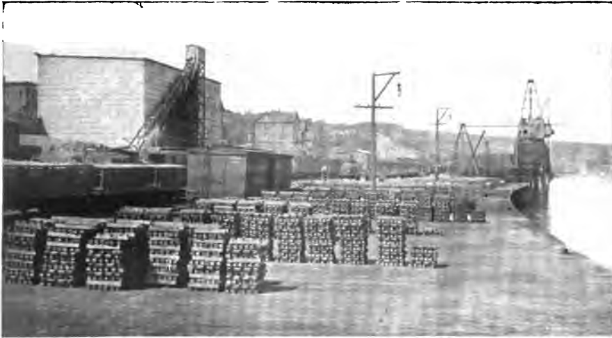
A. COPPER INGOTS ON DOCK AT HOUGHTON.
